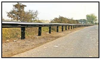
Aatmanirbhar Bharat has been made with the development of the world's first bamboo-made crash barrier, which has been installed on the Vani-Warora Highway in Vidarbh, Maharashtra. Additionally, it has also been accredited by the Indian Road Congress. The recycling value of the bamboo barrier is 50-70 per cent whereas that of steel barriers is 30-50 per cent.
